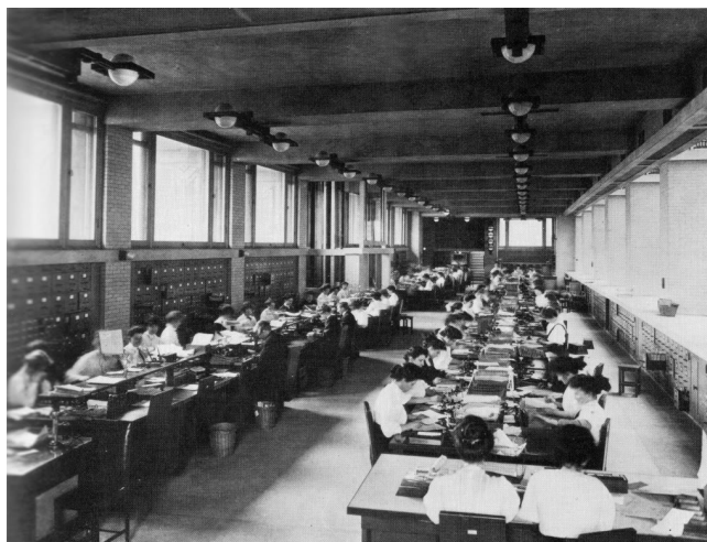
Obr. 26: Kanceláře Larkin Building II.
