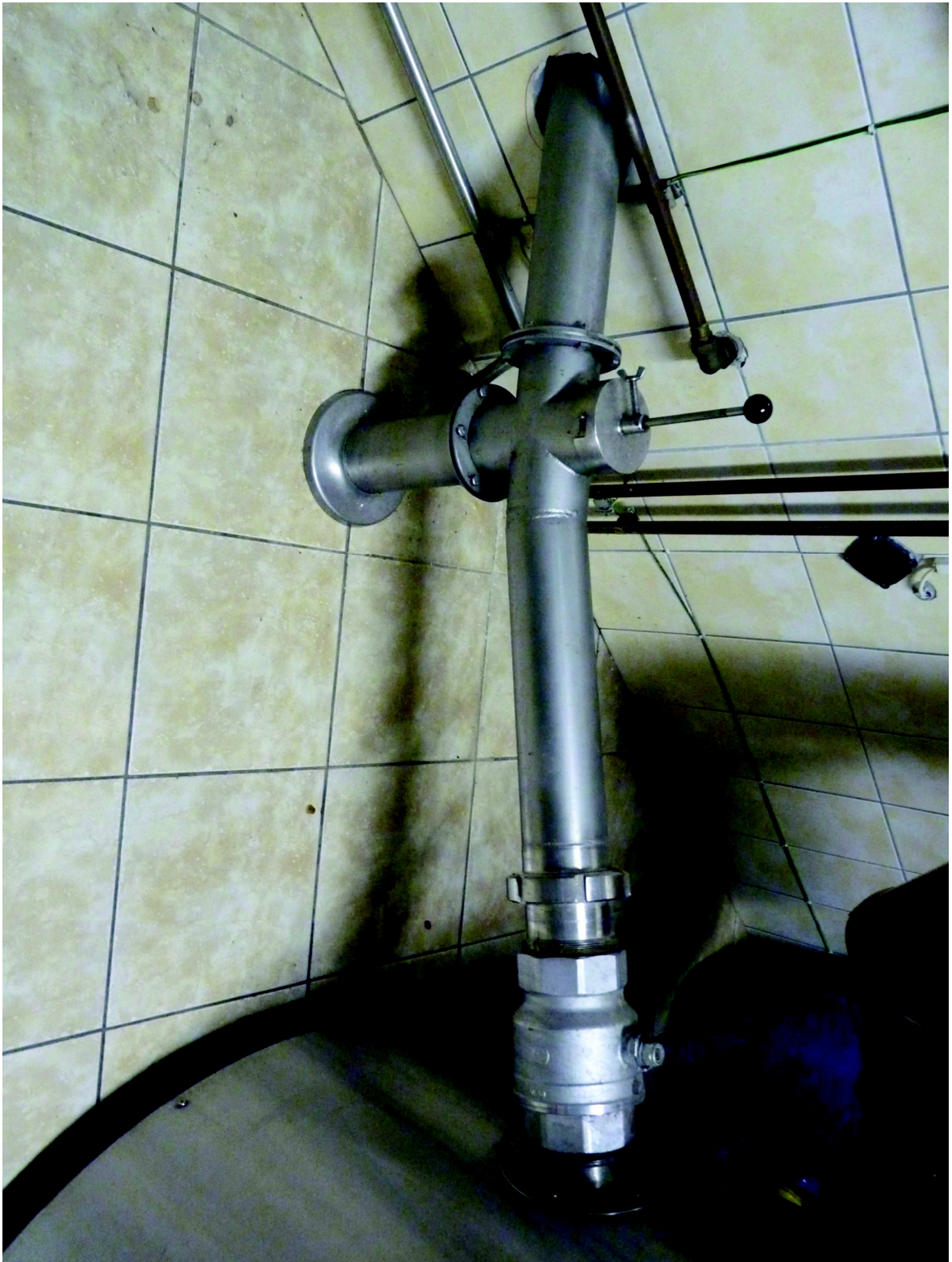
Pipe leading to the core-remover or sump, Appendix 6
