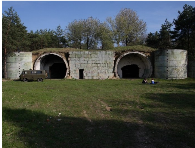
Photo 57: Special ammunition depot – Boží Dar u Milovic airport. [Source: Pho-57]
