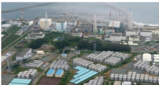
Photo 118: In the aerial photography of the Fukushima nuclear power plant from August 2013, the tanks with contaminated water can be seen. [Source: Pho-118]
