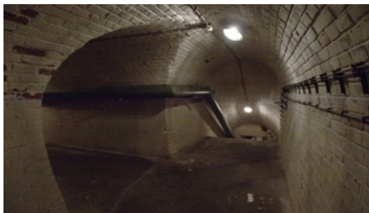
Photo 85: The civil protection shelters below the Spilberk Castle in Brno. [Source: Pho-85]
