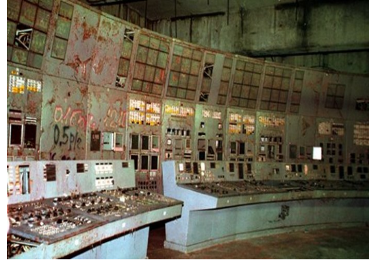
Photo 93: The control room of the Chernobyl nuclear power plant today. [Source: Pho-93]
