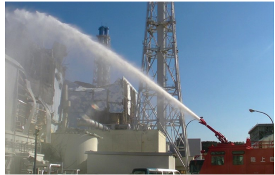
Photo 117: Adding water to the pool of Unit 3 of the Fukushima Daiichi nuclear power plant.
