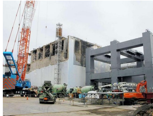
Photo 119: The construction of a new building where melted fuel rods will be stored.
