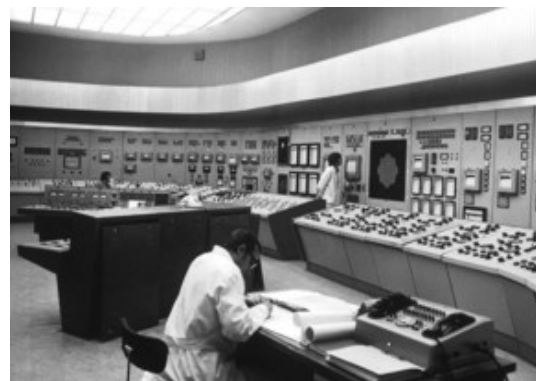
Figure 84: The main control room of the A-1 nuclear power plant. [Source: Fig-84]
