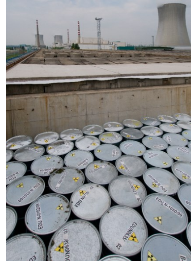
Figure 78: A vault with disposal drums at the Dukovany radioactive waste repository. [Source: Fig-78]
