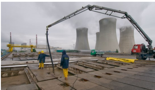
Figure 79: A vault with drums in the Dukovany radioactive waste repository. [Source: Fig-79]
