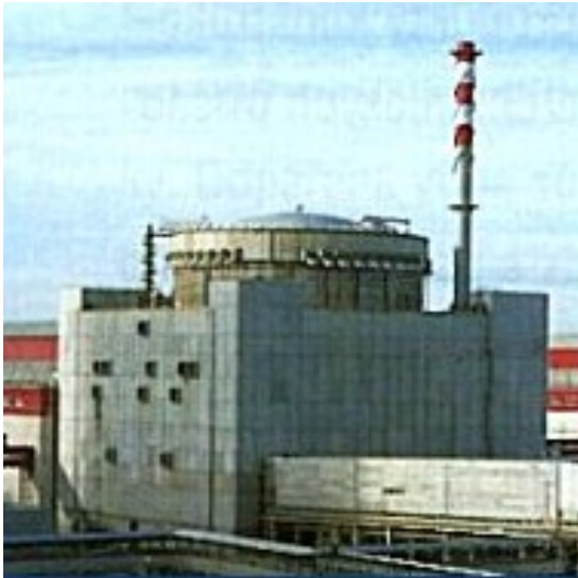
Figure 63: The containment with the reactor in the Temelin nuclear power plant. [Source: Fig-63]
