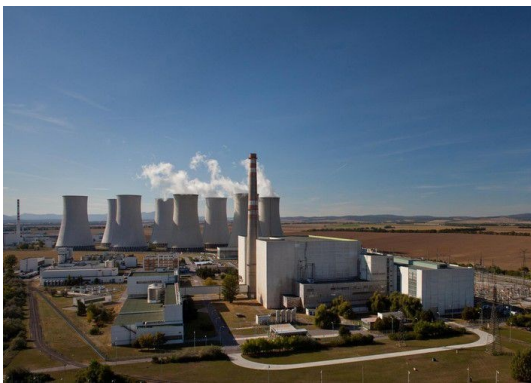
Figure 83: The A-1 nuclear power plant at Jaslovské Bohunice. [Source: Fig-83]
