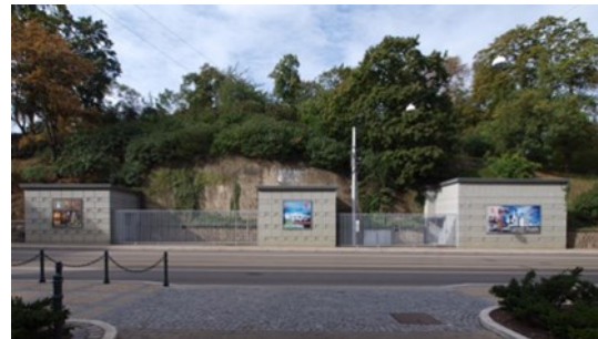
Photo 84: The civil protection shelters below the Spilberk Castle in Brno. [Source: Pho-84]
