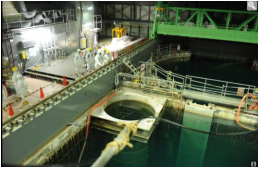
Photo 116: The water pool for storing used fuel in the Fukushima I power plant units.
