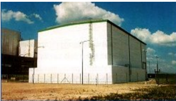
Figure 66: The storage of used fuel in the Dukovany nuclear power plant. [Source: Fig-66]
