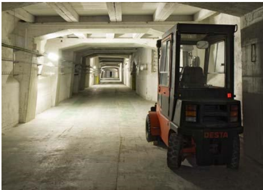
Figure 75: A tunnel in the Richard radioactive waste repository – Litoměřice. [Source: Fig-75]
