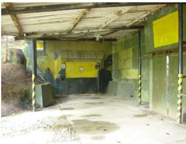
Photo 58: The JAVOR 51 nuclear ammunition depot in Míšov (Borovno). [Source: Pho-58]
