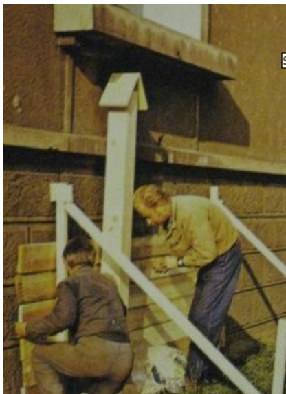
Figure 47: The construction of a chimney for an improvised shelter for up to 50 people (principle of gravity ventilation). [Source: Fig-47]
