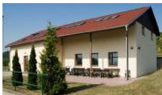
Figure 74: The administration building of the Richard radioactive waste repository. [Source: Fig-74]
