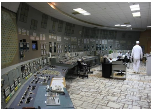
Photo 92: The control room of the Chernobyl nuclear power plant. [Source: Pho-92]
