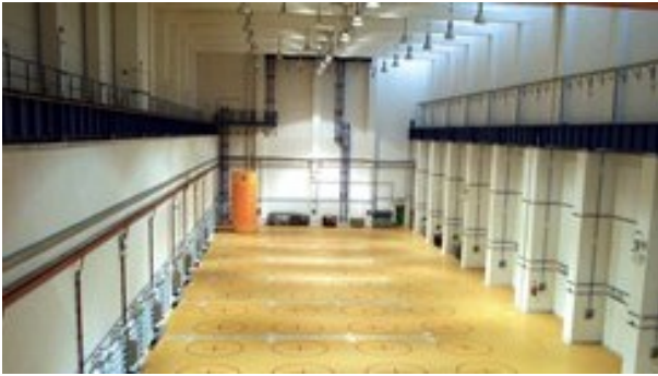
Figure 65: The storage of used fuel in the Temelin nuclear power plant. [Source: Fig-65]
