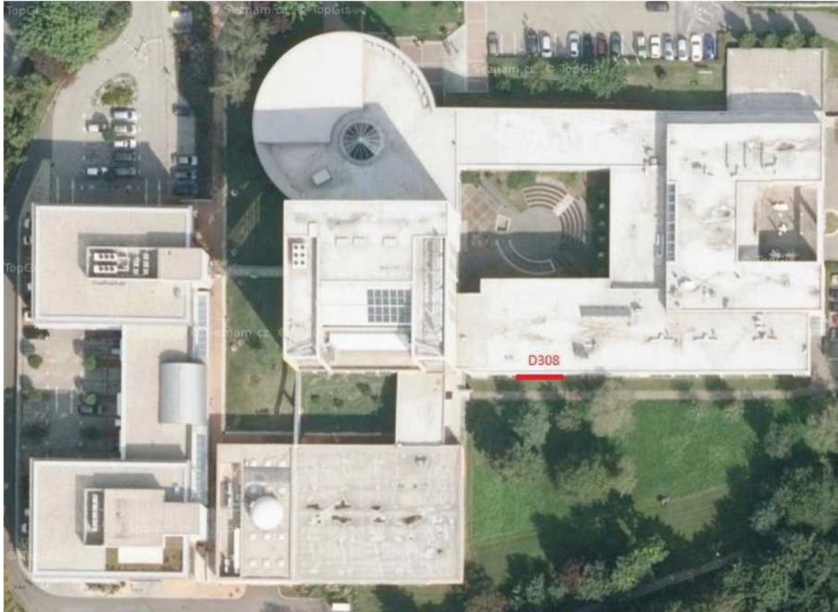
Fig. 22: FAI TBU Building (room D308 marked in red)
